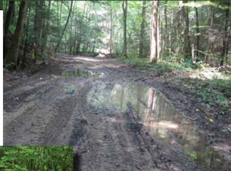
The accumulation of water on woodlands roads (above) creates erosion and access problems. If this is a persistent problem on your woodland roads then consider using geotextile fabric and gravel to address the issue.
