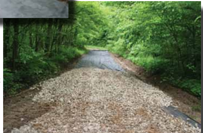
Spread the gravel (above) across all the fabric to a depth of four inches and then apply another two inches of smaller gravel as a final cap. The geotextile fabric should not be visible when you are finished.
