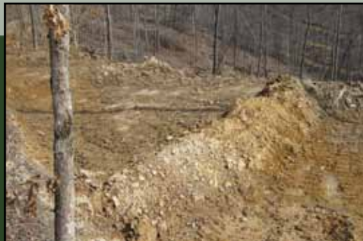
Photo courtesy: Daniel Bowker Best Management Practices (BMPs) such as the water bars shown in this image are designed to protect water quality during timber harvesting operations. BMPs significantly reduce the main water quality issue (sedimentation) associated with timber harvesting.
